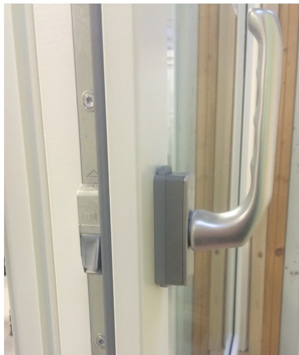
Fig 35a. Misuse inhibitor catch on tilt swing hardware
