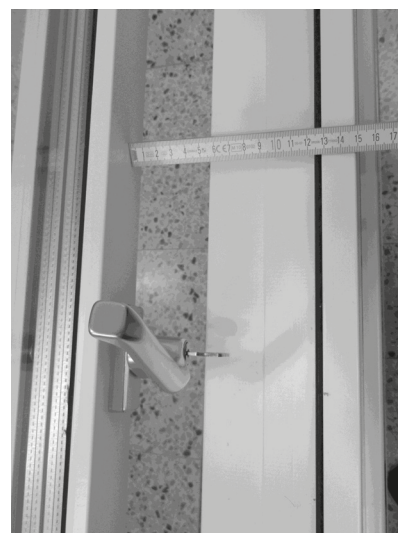
Fig 37. The fall safety device must lock the casement so that free movement does not exceed 10 cm.
