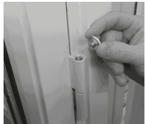
Fig 76. Removed cover for adjustable hinge.
