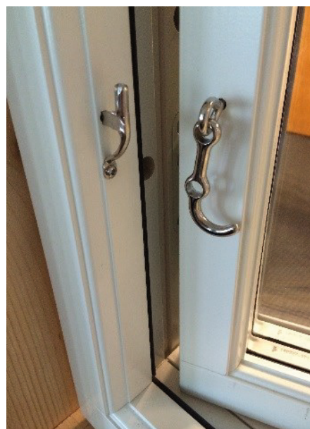
Fig 40. Installed airing hardware
