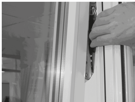
Fig 36. The catch for the hardware is moved towards the room to open the window.
