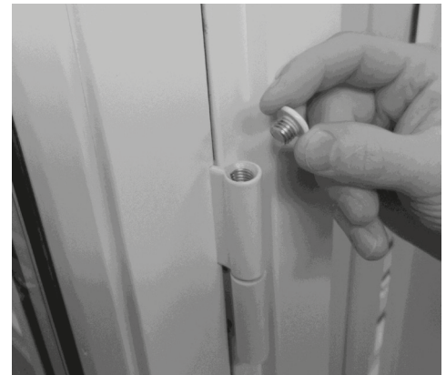
Fig 56. Removed cover for adjustable hinge.
