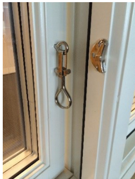
Fig 39. Installed lock and hook
