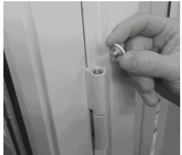
Fig 33. Removed cover for adjustable hinge.
