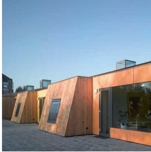
Built by 3BTEC Holzbau GmbH based in Ludwigsfelde, Germany
