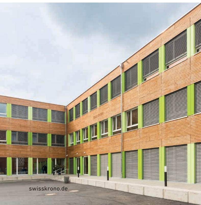
Built by ERNE AG Holzbau based in Aargau, Switzerland
