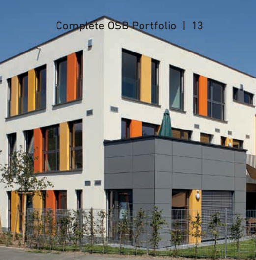
Built by Paul Riegel Foundation (HARIBO) in Bonn, Germany
